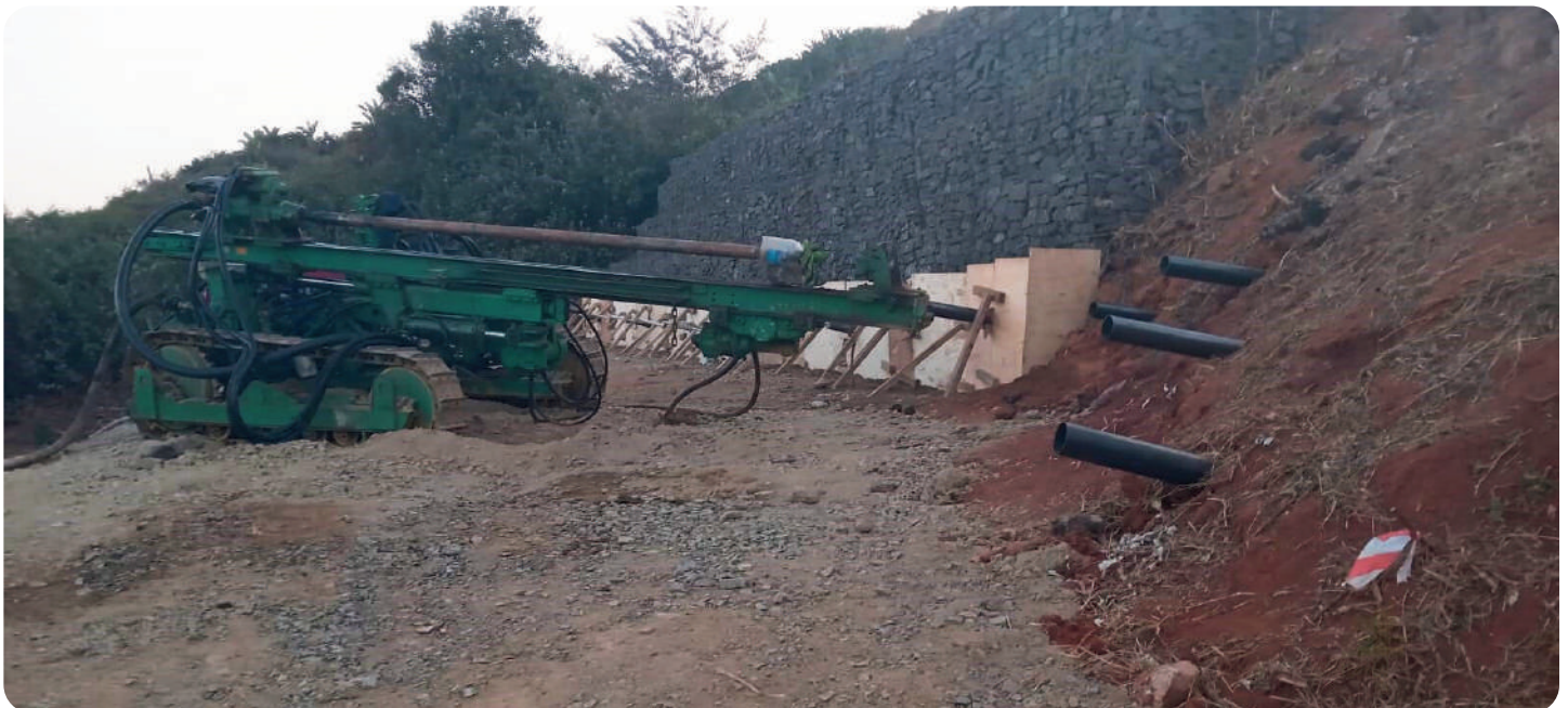
Soil Nailing into an Existing Gabion Retaining Structure
