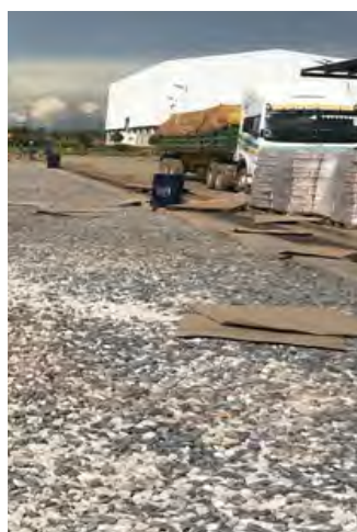
Figure 5: Complete Infiltration drain system with final rock fill layer complete.
